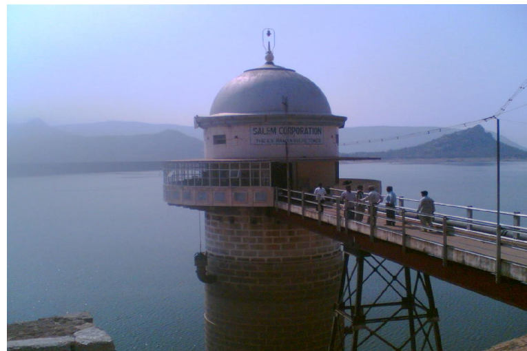
RAMAN INTAKE TOWER – METTUR SALEM SCHEME
